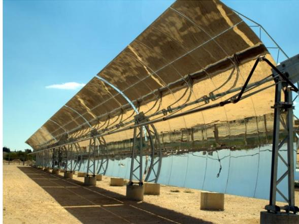
Figure 2: Parabolic trough
