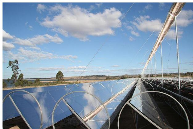
**Figure 4: Fresnel field of the SHP Company in Australia**
